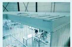
The modular construction system of ProCleanroom is flexible, portable and can be easily expanded. ProCleanroom provides hardwall cleanrooms, softwall cleanrooms and mini environments.
